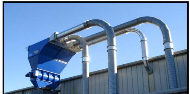
The existing Separation plant above the Baler was replaced with an Airmec's Separator and Rotary Valve system which was sized to accommodate their latest requirements. Existing ductwork was remodelled to allow smooth waste transfer into the Separator.
